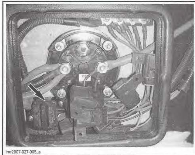
TYPICAL - REAR OF MAIN BATTERY CUT-OFF SWITCH
