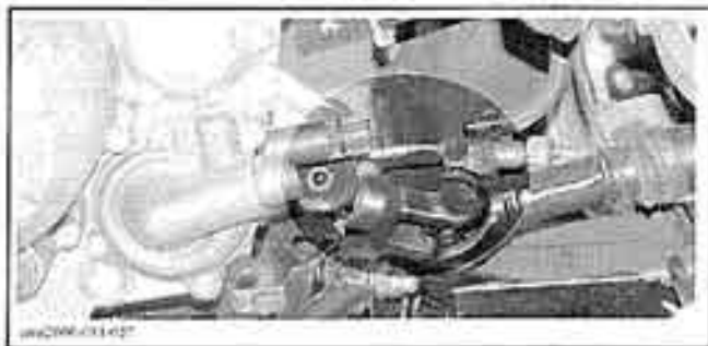
LIFT ENGINE AND DISCONNECT THE FRONT PROPELLER SHAFT FROM ENGINE
